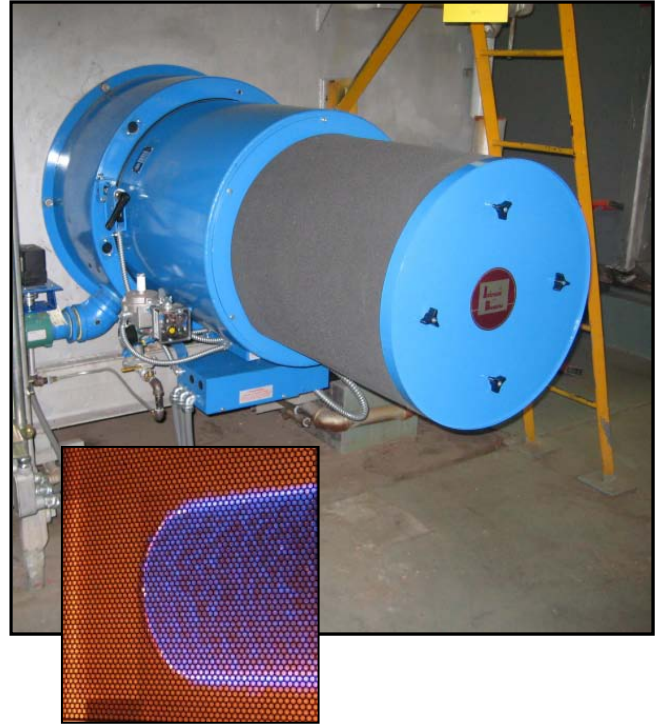
Model NM300A firing a 300 HP watertube boiler at sub-9 ppm NOx.
